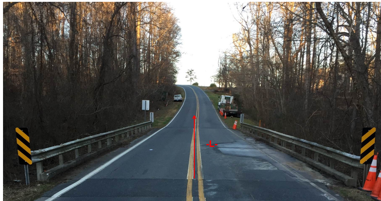
View Looking North along -L- from End Bent 1
