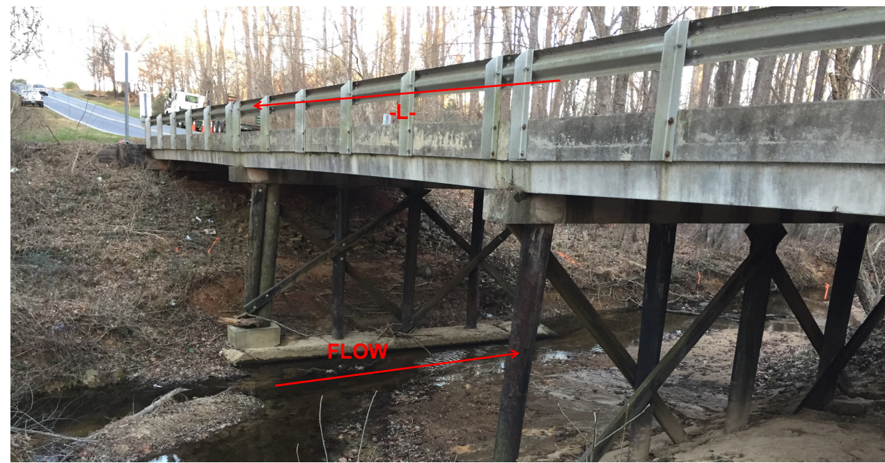
Profile of Existing Bridge from West of End Bent No. 1
